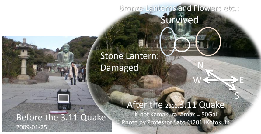
Figure 8. Damage example by the 2011.3.11 Tohoku earthquake
