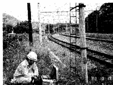
View of the microtremor measurement along JR line using PIC87
