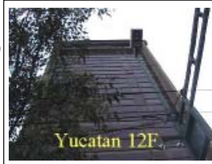
Fig.1 External appearance of measured building
