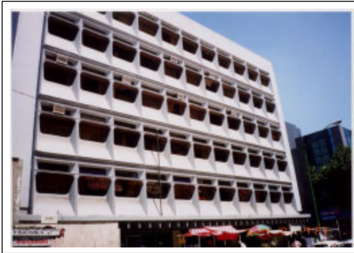
Fig.1 External appearance of measured building
