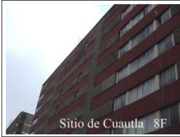
Fig.1 External appearance of measured building
