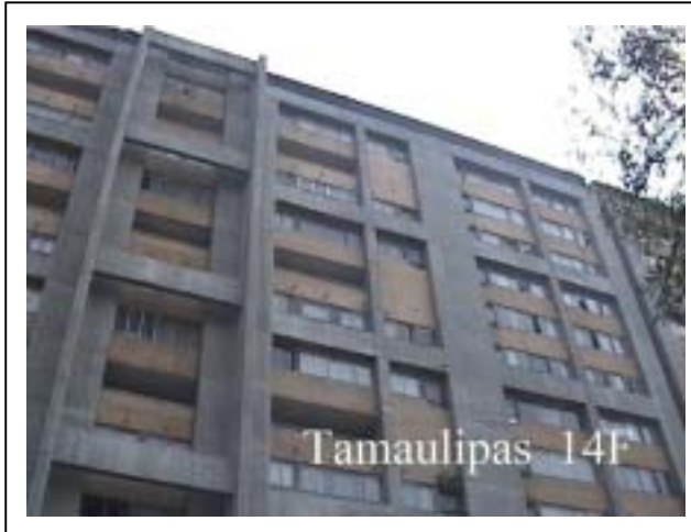
Fig.1 External appearance of measured building
