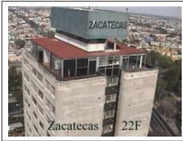
Fig.1 External appearance of measured building
