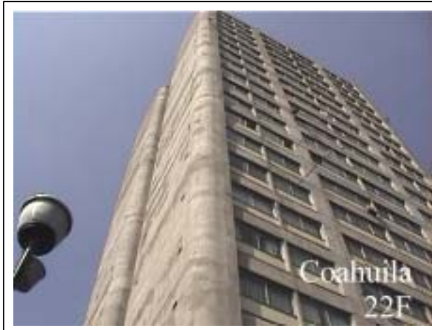
Fig.1 External appearance of measured building
