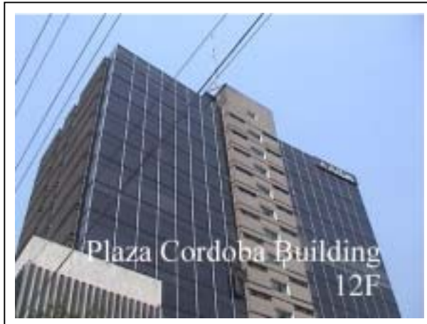
Fig.1 External appearance of measured building
